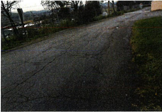
Asphalt damage/potholes
