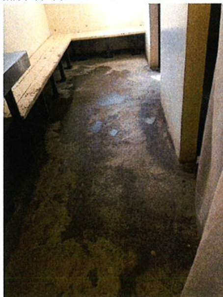
Poor drainage in shower area
